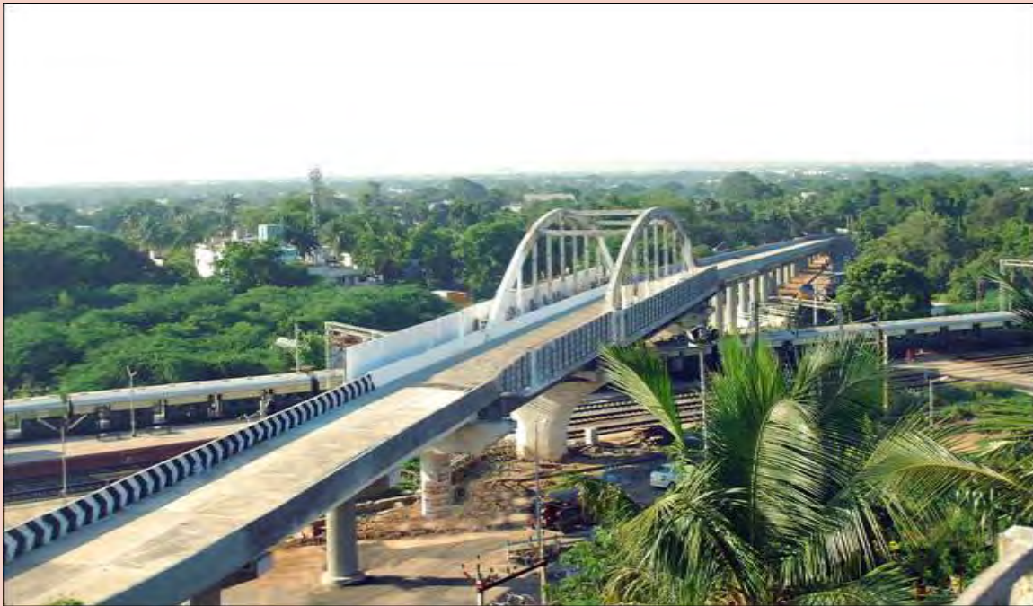
Railway Over Bridge at Pallavaram, Chennai inaugurated by the Hon'ble Chief Minister on 09.10.2012.
