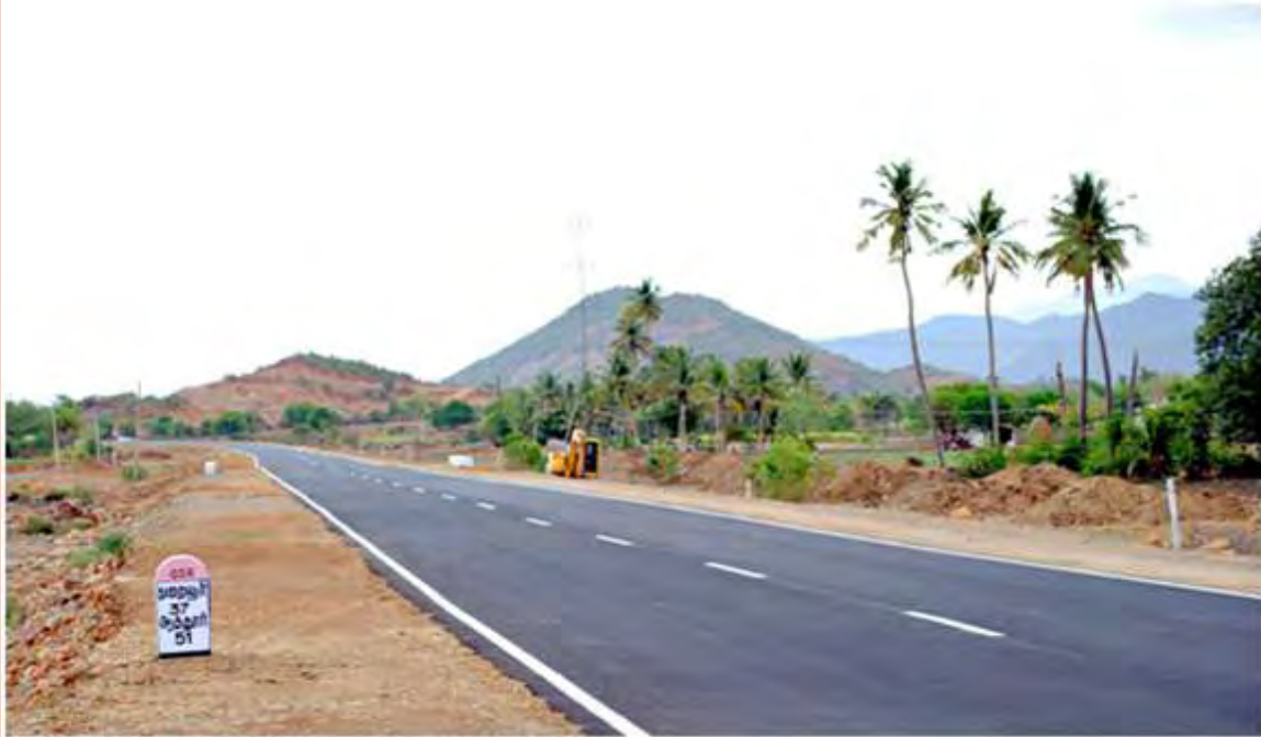
Perambalur Bypass inaugurated by the Hon'ble Chief Minister on 09.10.2012.
