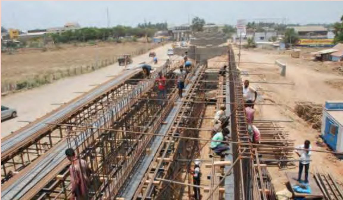
Ongoing Railway Over Bridge work at Eachanari, Coimbatore.
