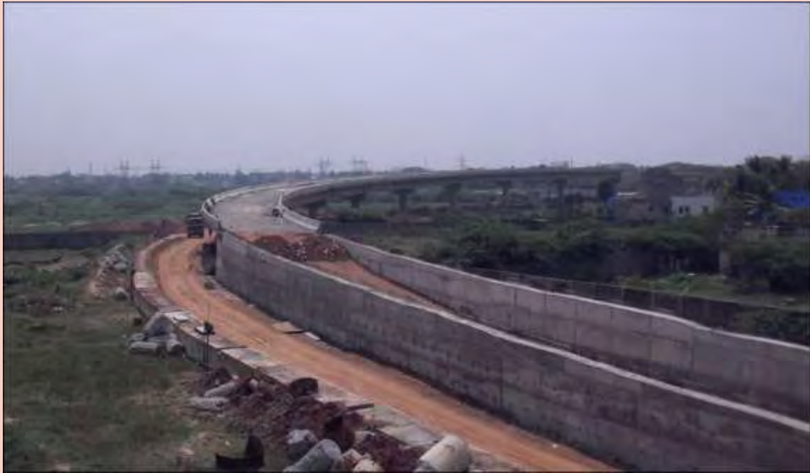
Ongoing Railway Over Bridge work at Pattaravakkam, Chennai.
