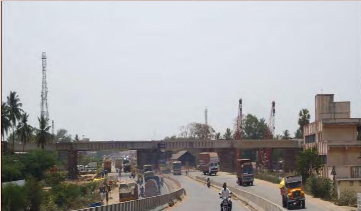
Ongoing interchange work at Nazarathpet (NH 4) on Chennai Outer Ring Road.
