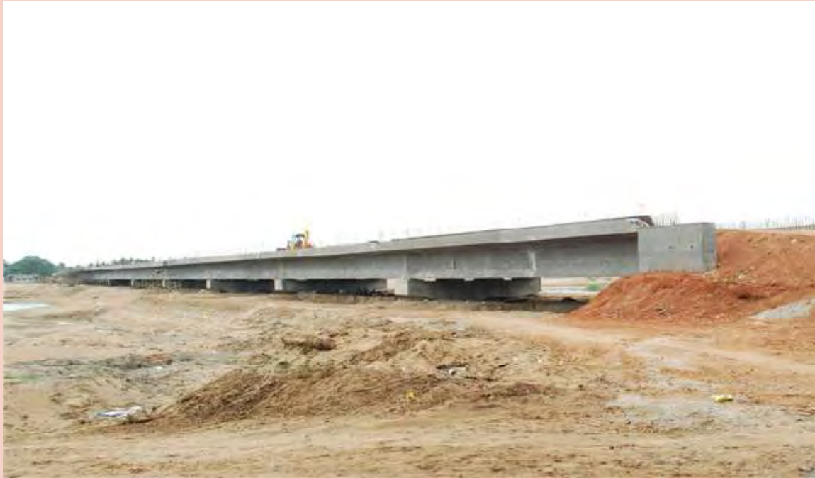
Ongoing High Level Bridge work across Cauvery at Thirukattupalli, Thanjavur District
