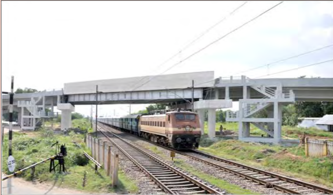
Railway Over Bridge at Thiruvallur, Vellore District inaugurated by the Hon'ble Chief Minister on 09.10.2012.
