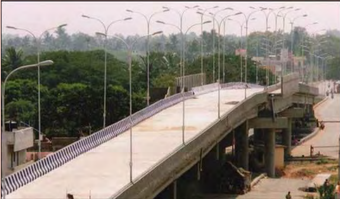
Railway Over Bridge at Pakkam, Maduranthagam inaugurated by the Hon'ble Chief Minister on 30.01.2013.
