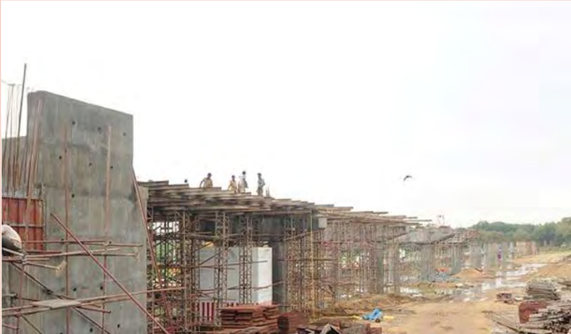
Ongoing High Level Bridge work on Nazerath – Eral road, Tuticorin District
