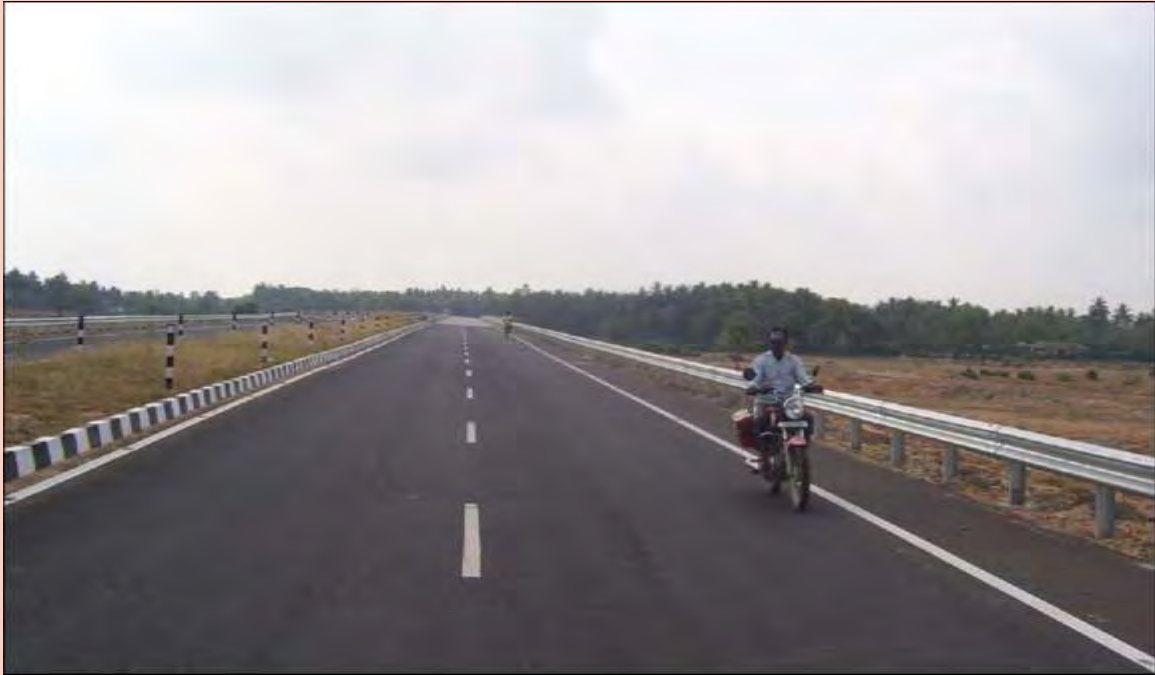
Ongoing Bypass work at Kancheepuram
