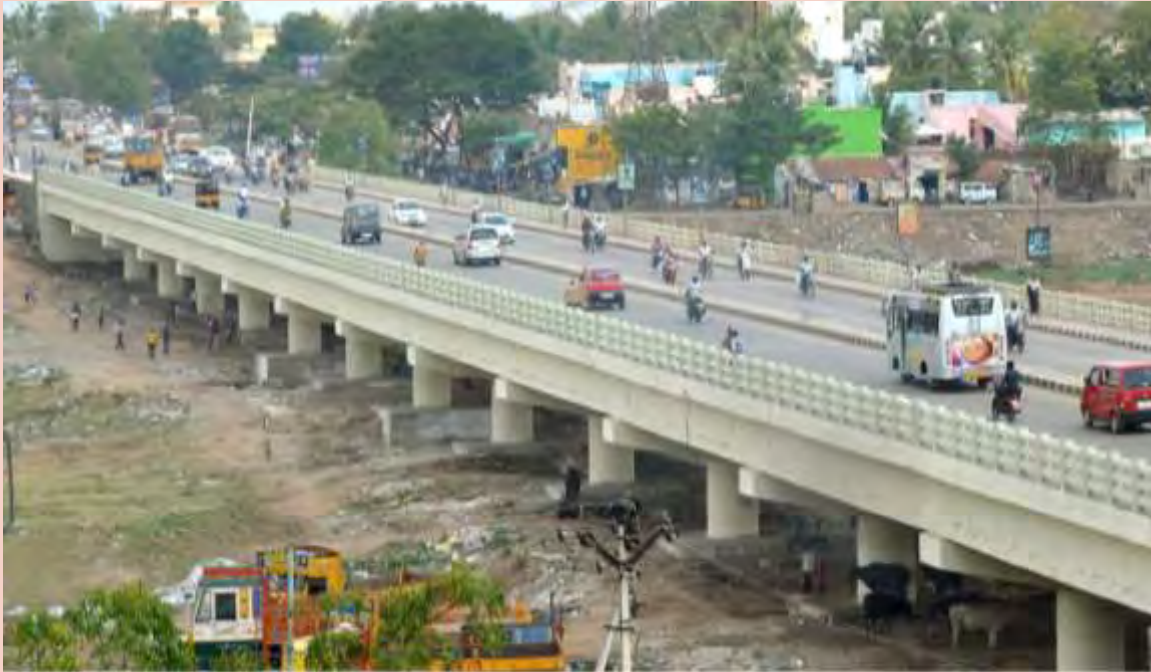
High Level Bridge across Vaigai at Madurai inaugurated by the Hon'ble Chief Minister on 09.10.2012.
