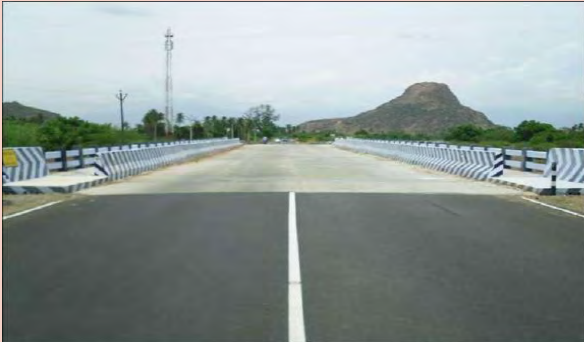
Bridge on Madurai – Cochin Road near Thimmarasanaickanur inaugurated by the Hon'ble Chief Minister on 09.10.2012
