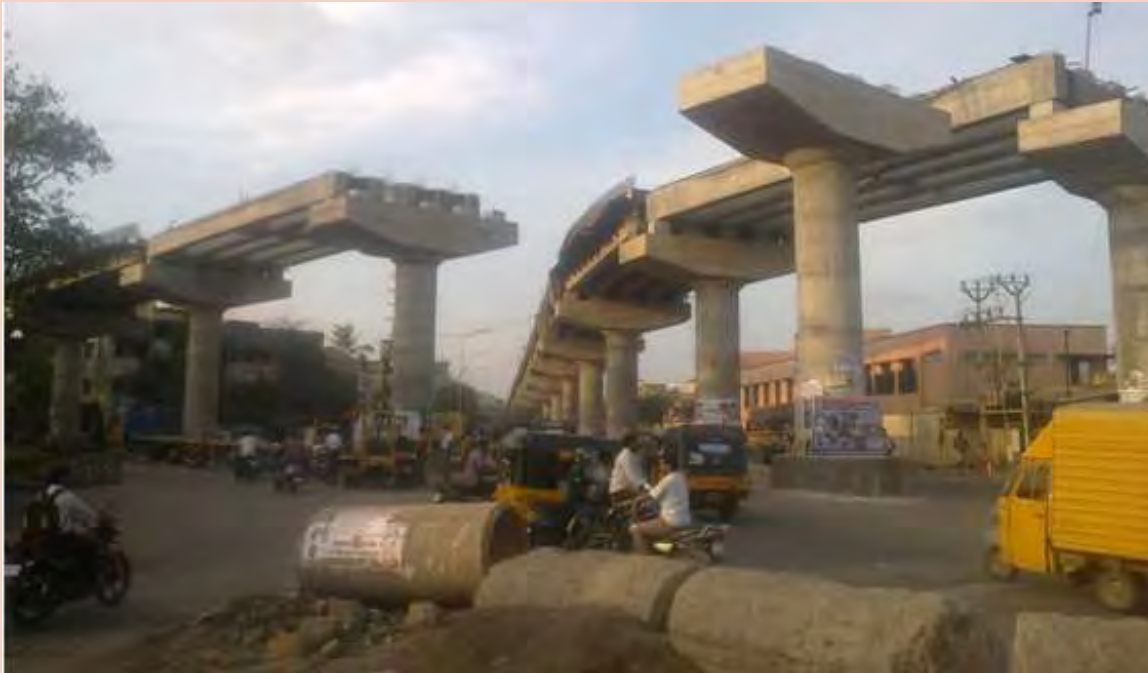
Ongoing Railway Over Bridge work at Vyasarpadi, Chennai.
