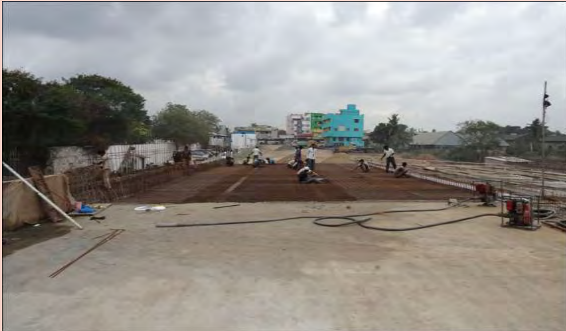
Ongoing River Bridge work across Couam River at Mogappair, Chennai.
