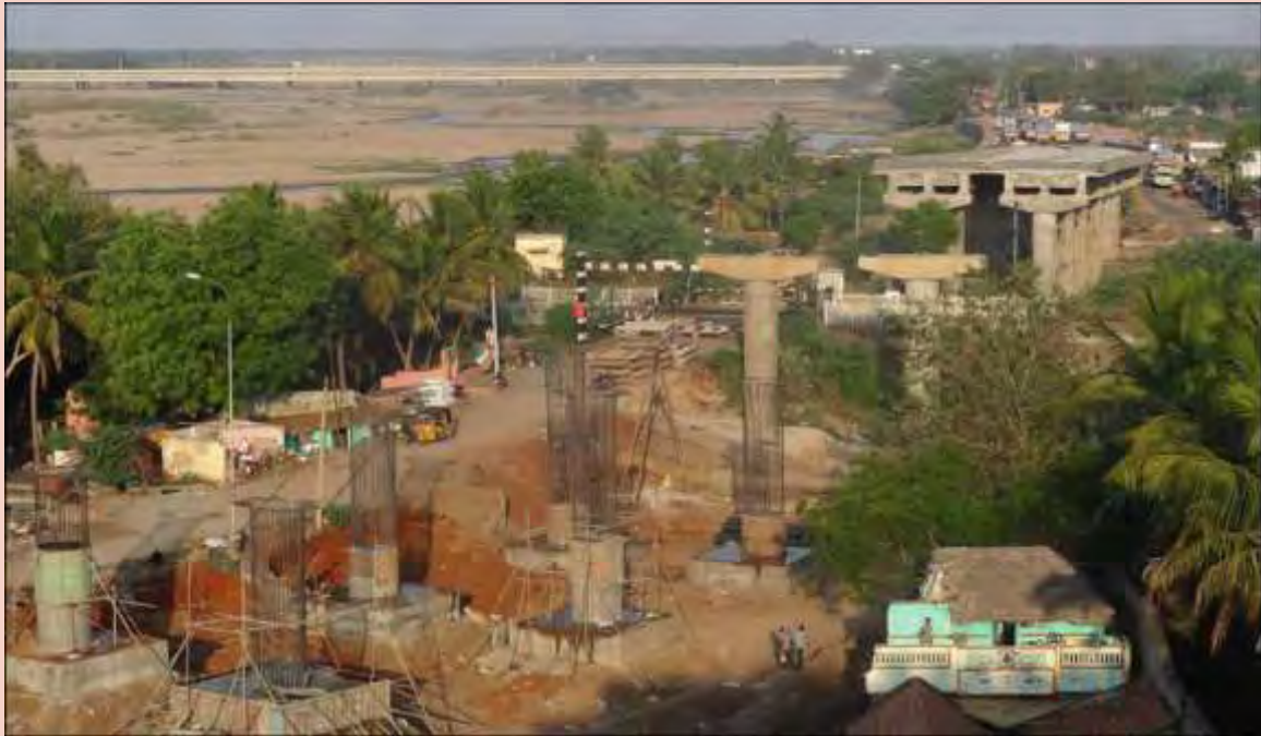
Ongoing Railway Over Bridge work near Kollidam River, at Srirangam, Trichy
