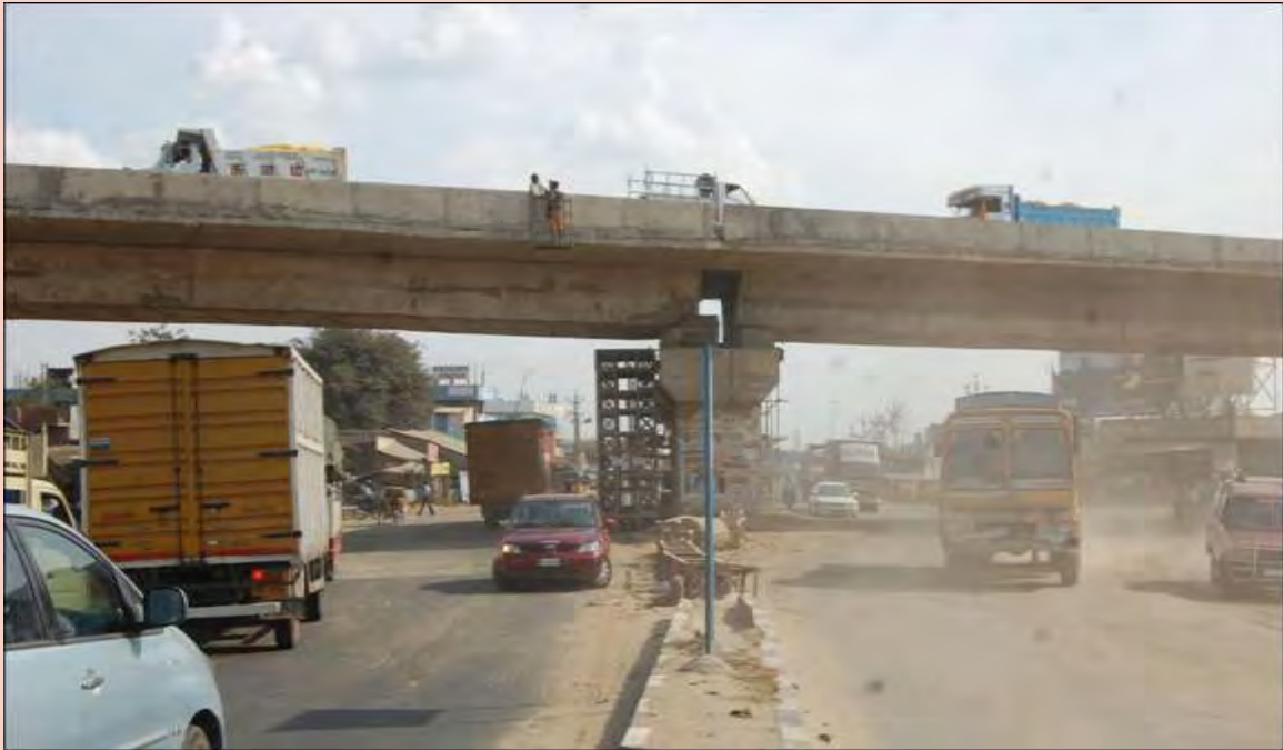
Ongoing Grade Separator work at Oragadam under the Industrial Corridor Project.
