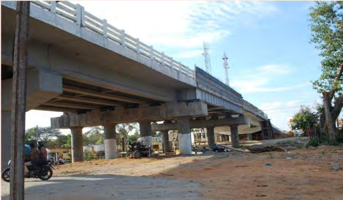
Completed Railway Over Bridge at Coolipalayam, Tiruppur
