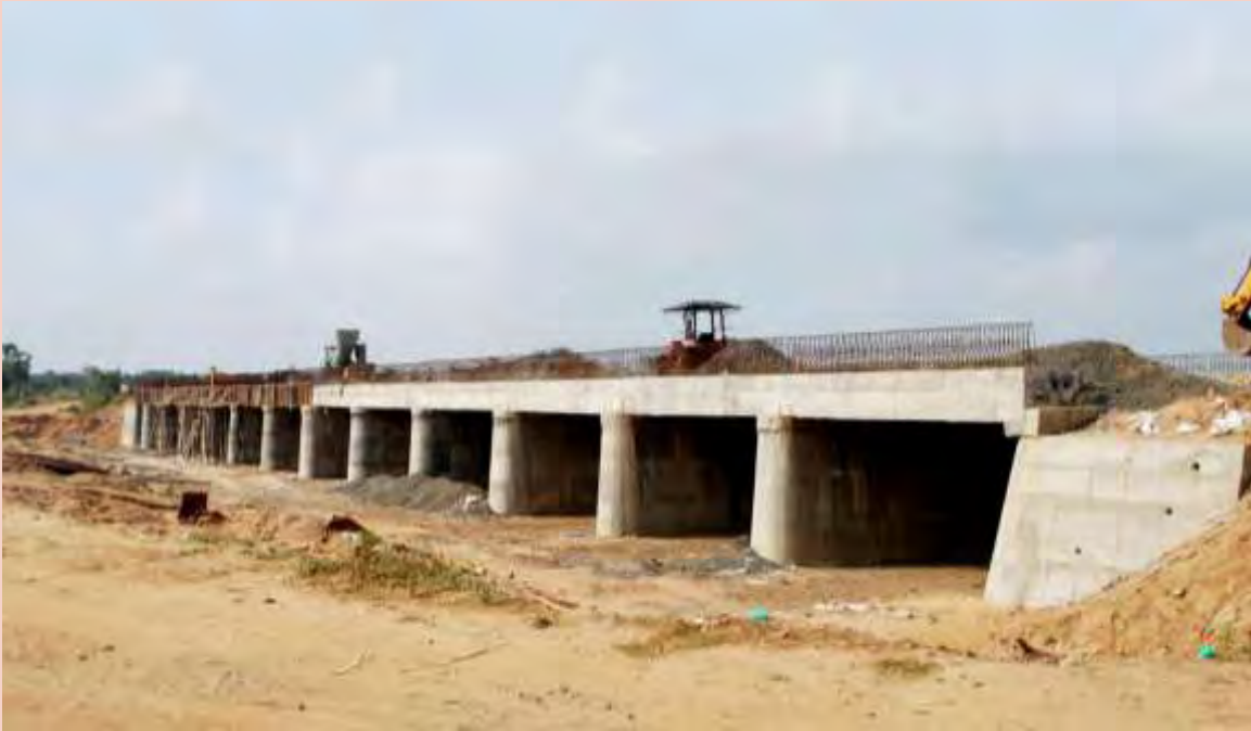
Ongoing High Level Bridge work on Pudukottai – Embal Road, Pudukottai District
