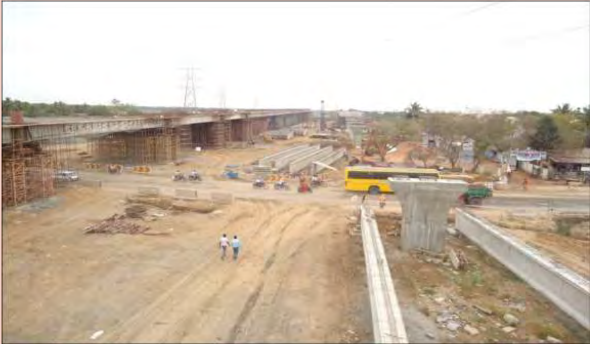
Ongoing interchange work at Nemilicherry (NH 205) on Chennai Outer Ring Road.
