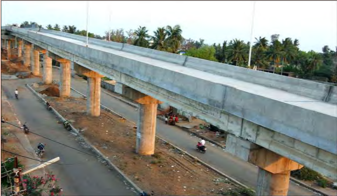
Completed Railway Over Bridge work at Virudhachalam.
