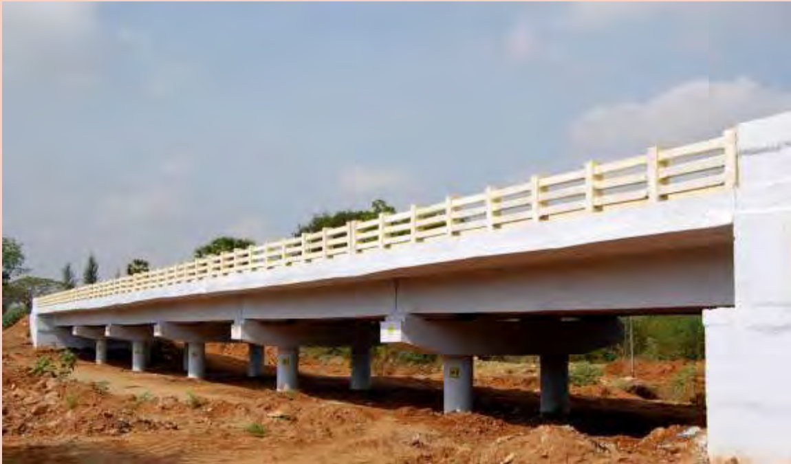
High Level Bridge work on Maruthupatti – SS Kottai road, Sivagangai District inaugurated by the Hon'ble Chief Minsiter on 30.01.2013
