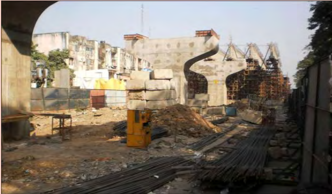
Ongoing Grade Separator work at Thirumangalam, Chennai.
