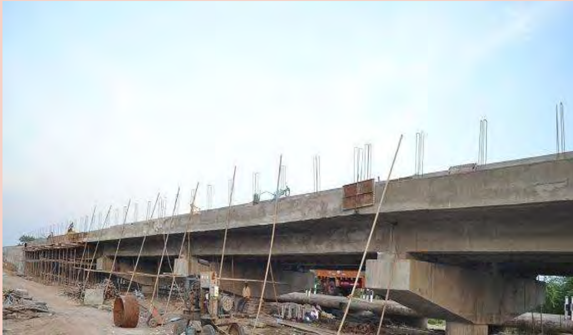
Ongoing High Level Bridge work on Srivilliputhur – Parthibanur Road, Virudhunagar District
