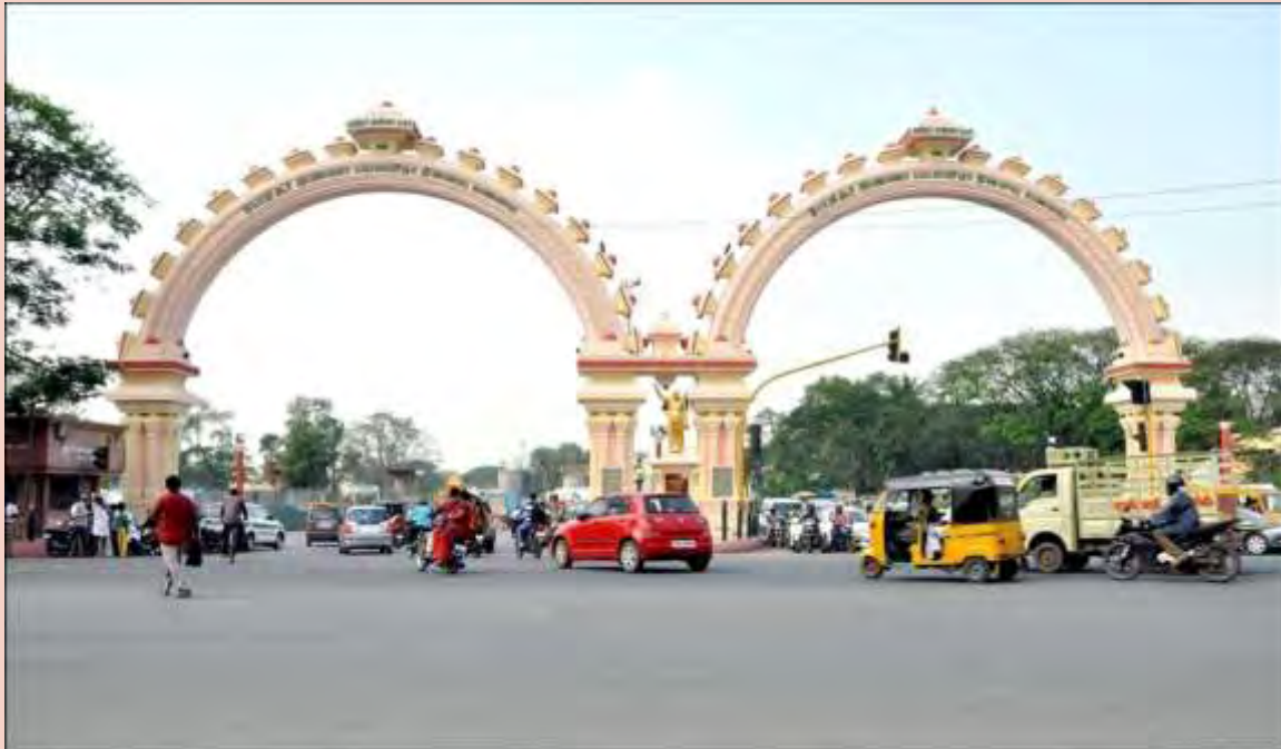
The restored Anna Arch opened for traffic on 04.01.2013
