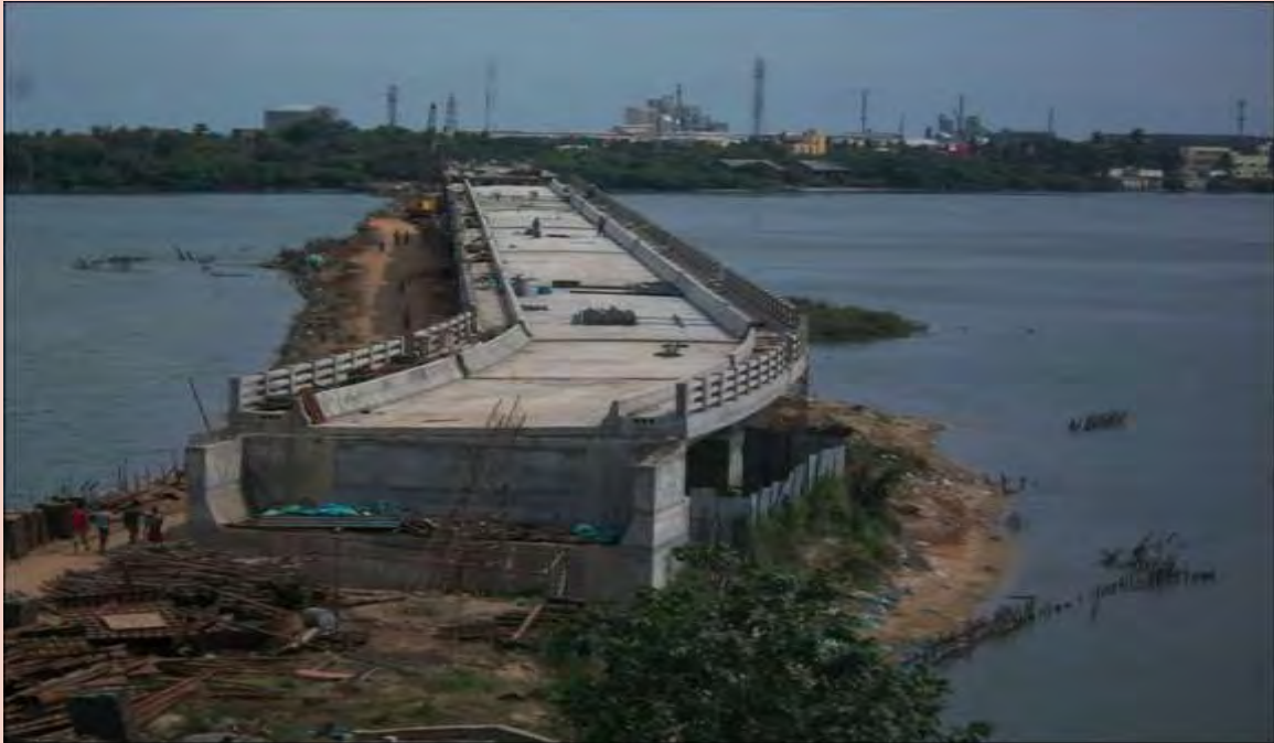
Ongoing High Level Bridge work at Ennore Creek, Chennai.
