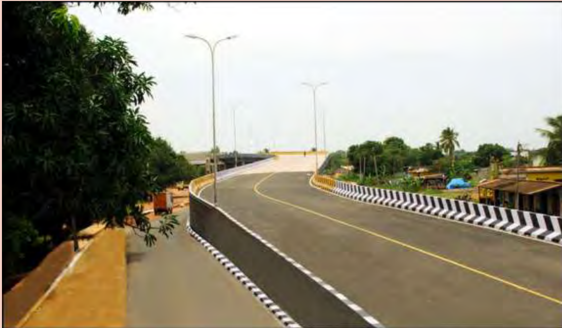
Railway Over Bridge at Gummidipoondi inaugurated by the Hon'ble Chief Minister on 09.10.2012.
