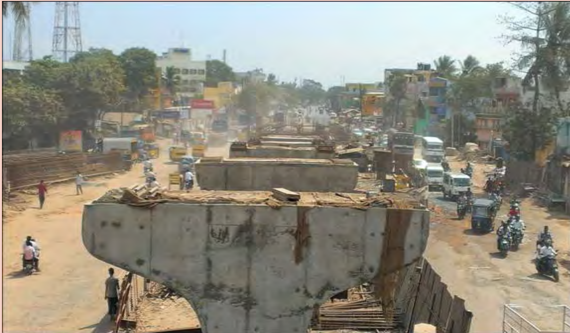
Ongoing Grade Separator work at Moolakadai, Chennai.
