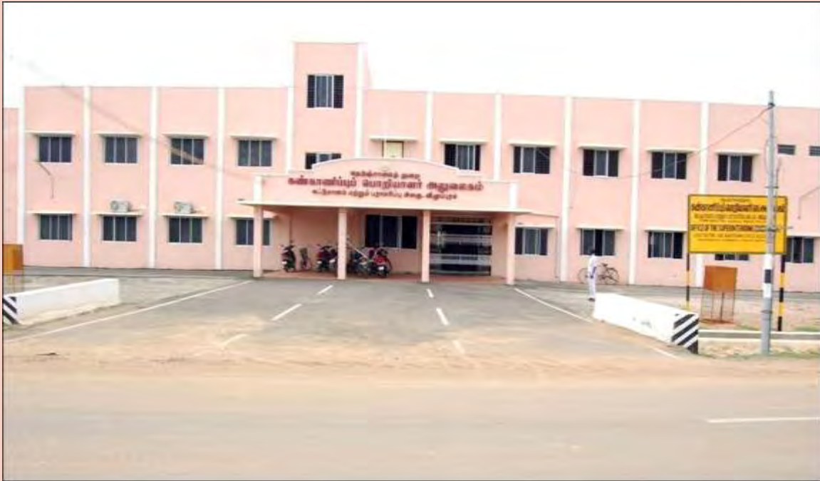
Highways Office Complex at Villupuram inaugurated by the Hon'ble Chief Minister on 09.10.2012.
