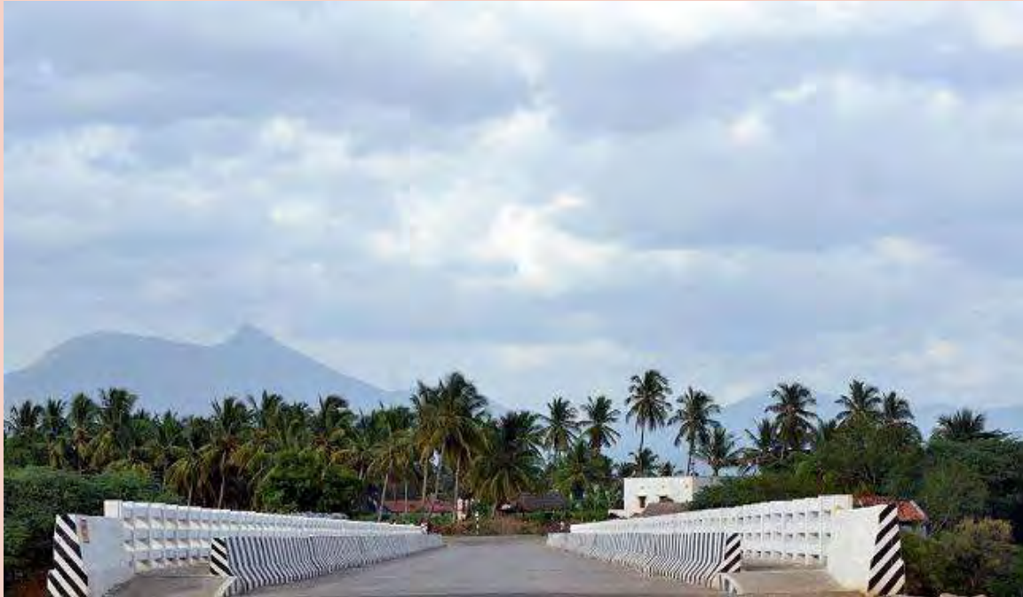
Bridge on Mudukanthurai - Erankattur Road, Erode District inaugurated by Hon'ble Chief Minister on 09.10.2012
