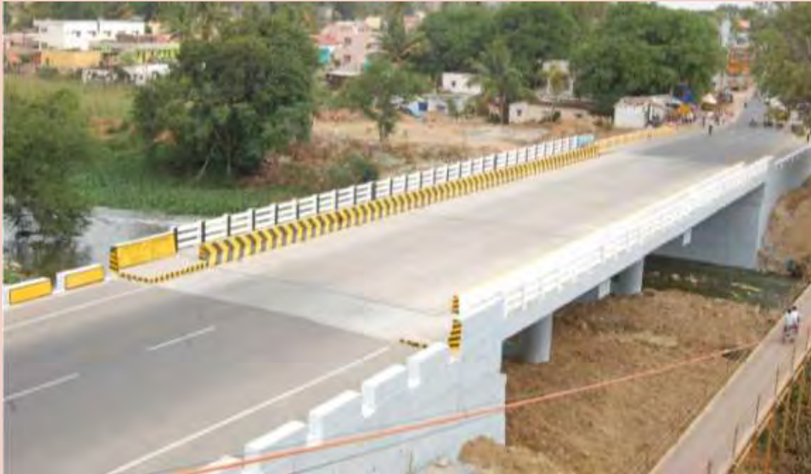
High Level Bridge at Paagalur, Krishnagiri District inaugurated by the Hon'ble Chief Minister on 09.10.2012.
