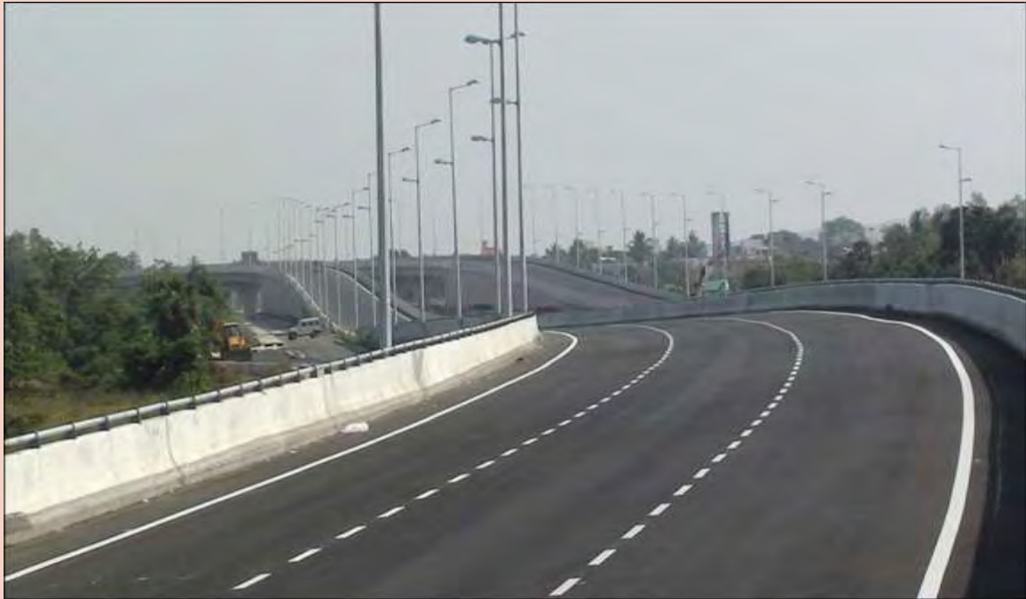
Flyover near Vandalur Tank on Chennai Outer Ring Road.
