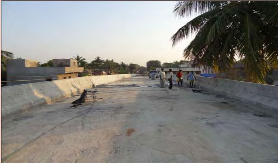
Ongoing Railway Over Bridge work at Veppampattu, Chennai.
