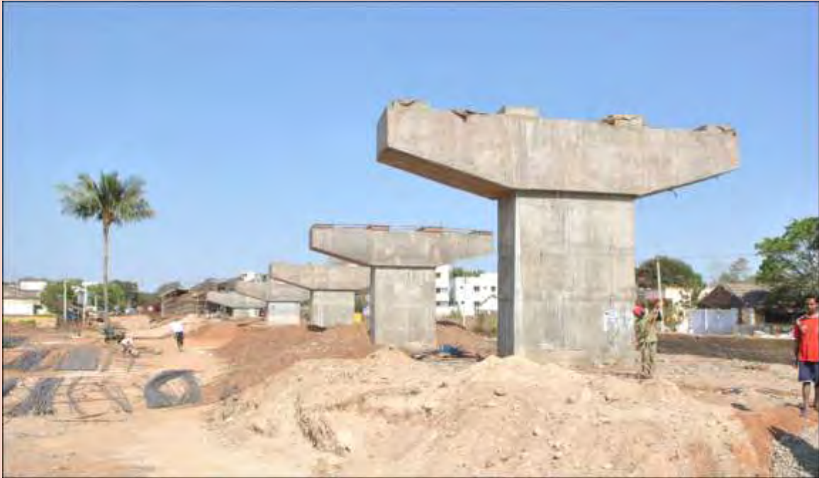
Ongoing Railway Over Bridge work at Manaparai, Trichy
